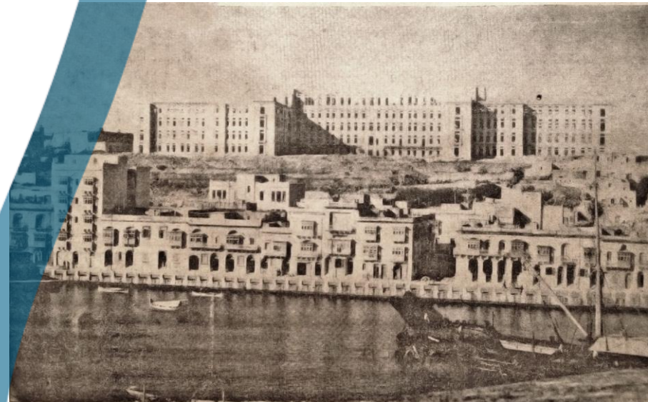
Building of St. Luke's hospital nearing completion, late 1930s
